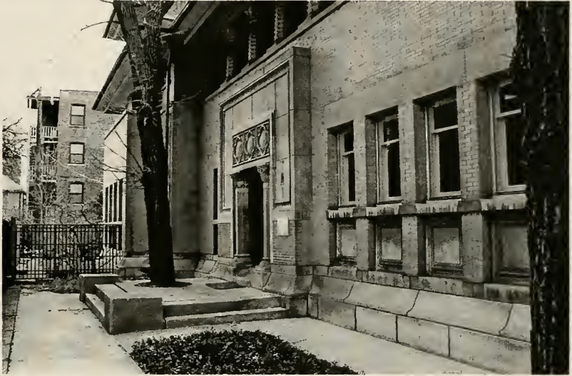
Figure 1.2 Entrance to the Heller House, South elevation. The loggia is visible on the second level. Photograph by the author, 1999.
